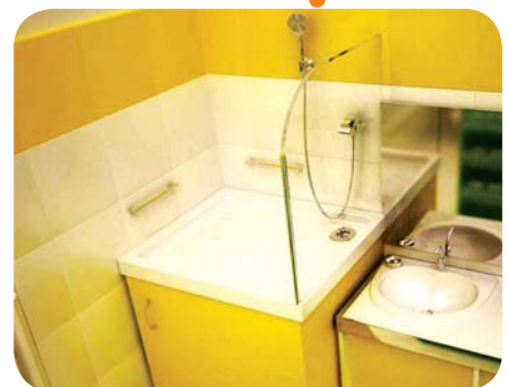
Shower for children (Made with handle for child and placed higher for teacher to clean children)
